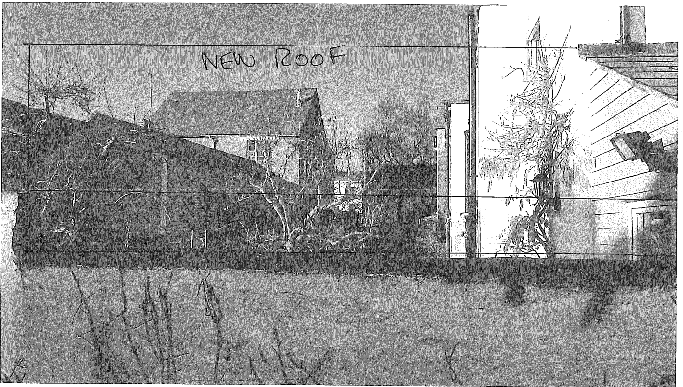
fig 2 View from my back yard with new roof and wall added.
